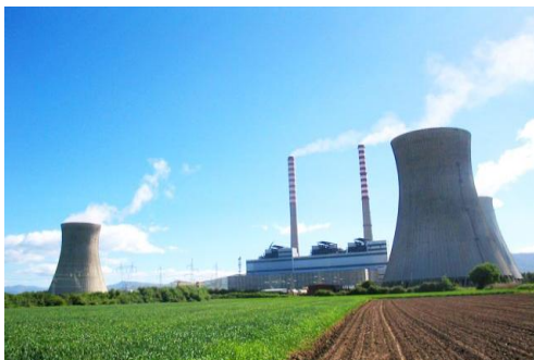
REK Bitola - Mining and Energy Combine
